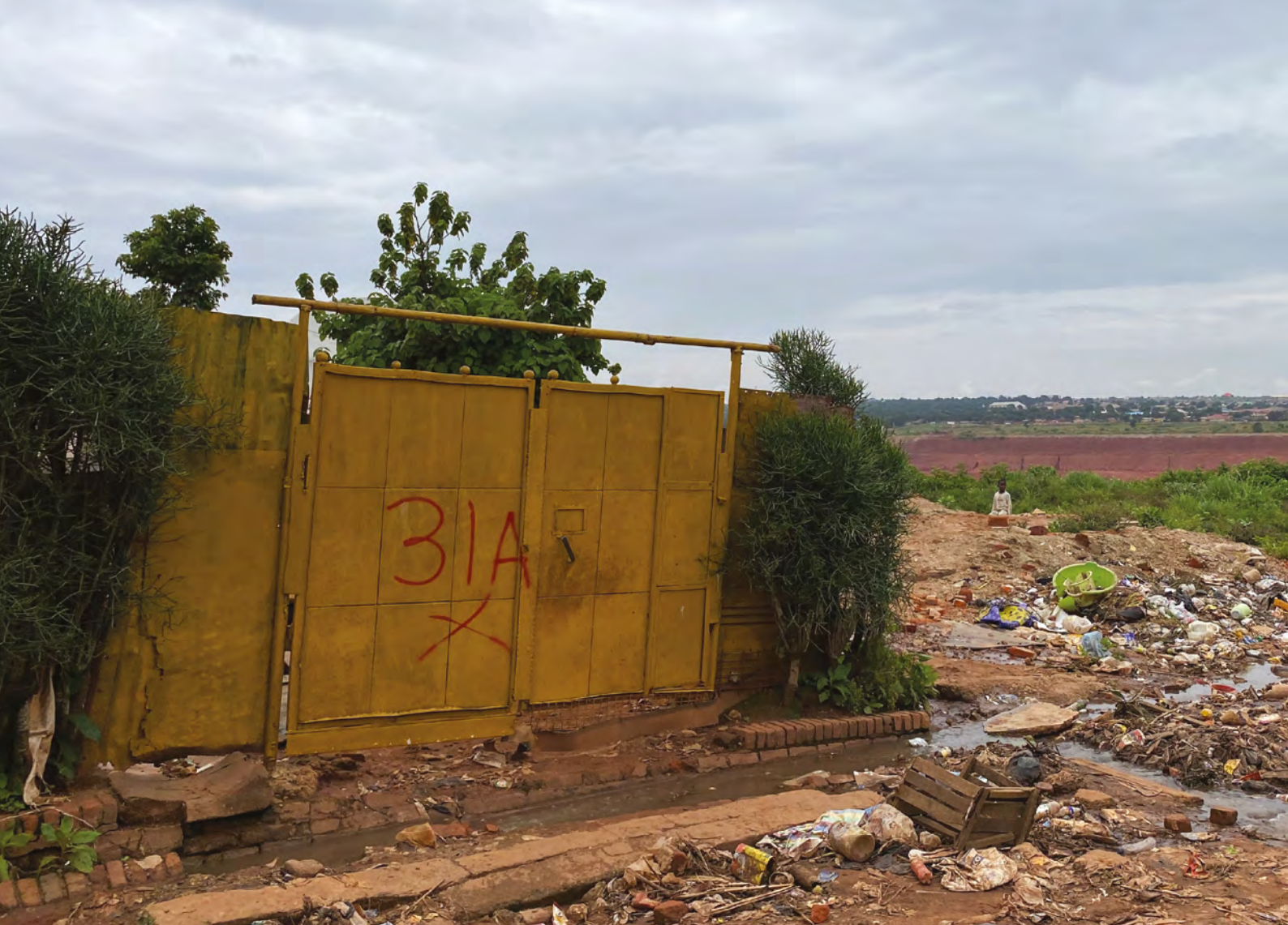
© ↑ House marked for eviction in Kolwezi, DRC, on the edge of the open-pit Kolwezi copper and cobalt mine © Amnesty International September 2022
